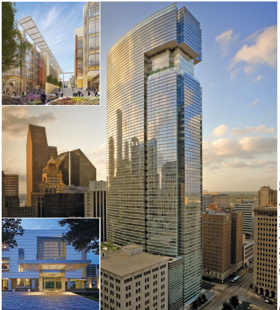
BG Group Place , headquarters for the international natural gas company, was completed in February 2011 in downtown Houston. The design by Pickard Chilton recently won an award from AIA New England. Other recent energy firm headquarters projects have come from ExxonMobil (upper left inset) and ConocoPhillips (lower left inset).
